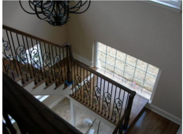
Figure 10 – Glass in stair landing
