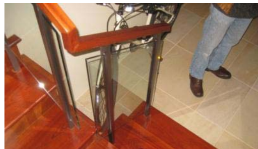
Figure 8 – Laminated glass in guard infill
