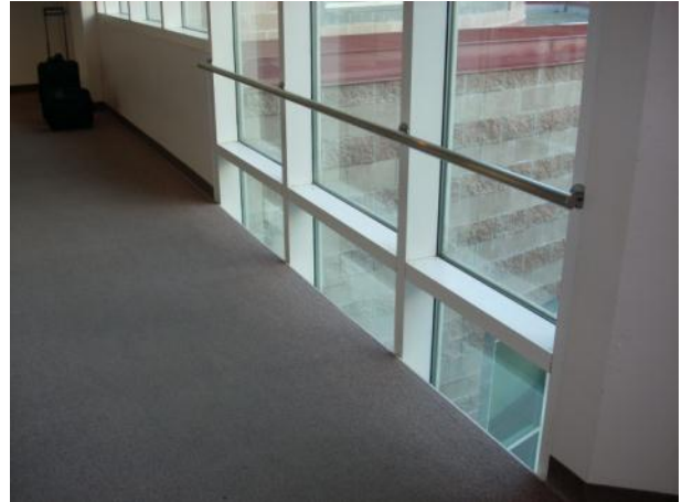
Figure 7 – Protective bar in front of window
