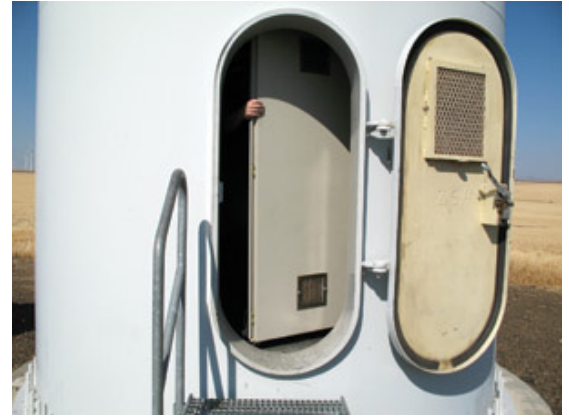
Figure 8. This is a clear violation of the access and egress requirements of the NEC. The Code requires a “continuous and unobstructed way of egress travel.”
