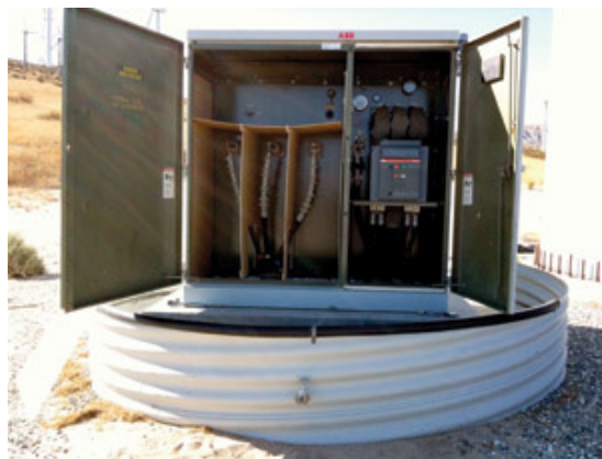
Figure 9. Does this say adequate working space to you? This containment vessel is both a shock and trip hazard. According to 110.26(A)(3) of the NEC, “... The work space shall be clear and extend from the grade...”.
