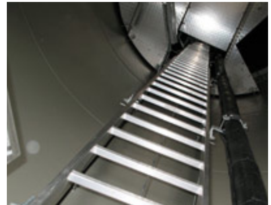
Figure 5. Does this strain relief fastener arrangement for this 34.5kV cable meet code requirements?
