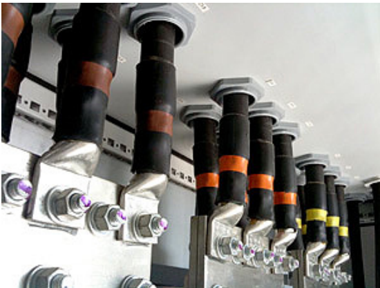
Figure 11. The lack of slotting or larger openings with insulating walls will induce circulating currents on the ferrous metal enclosure wall that could potentially produce insulation damaging heating.
